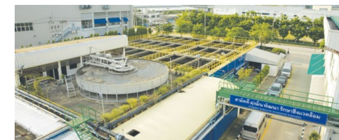
24 MLD Wastewater Treatment Plant in Amata Industrial Estate Chonburi, Thailand
