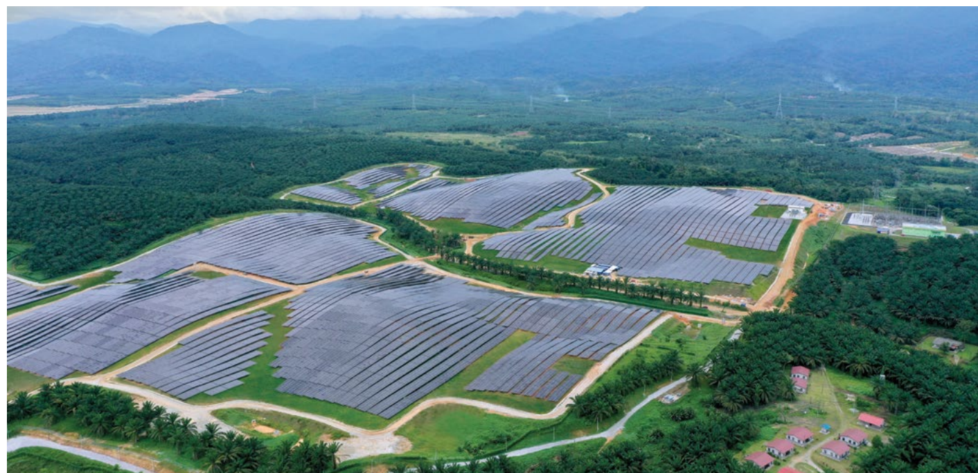
Large Scale Solar Farm ("LSS4") located at Bidor, Perak
